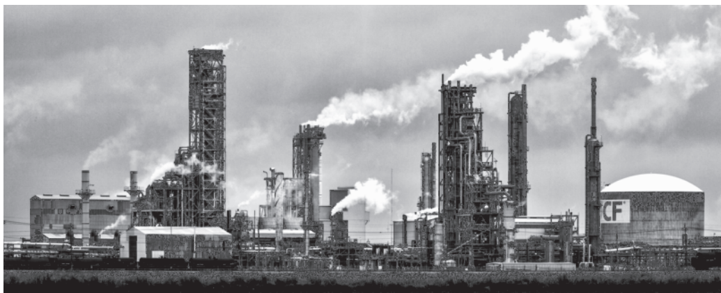
Left: The company's facility in Donaldsonville, Louisiana, is the largest nitrogen manufacturing complex in North America.
